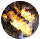
Fakel Burner Inspection
