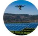
Photovoltaic Power Plants
